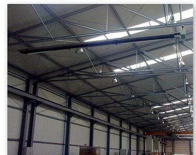
When considering the choice of a new energy-efficient heating system for halls, warehouses, workshops or greenhouses, we should definitely consider gas-powered radiant heating. State-of-the-art heating systems for large-space buildings are increasingly based on gas radiant heaters.
